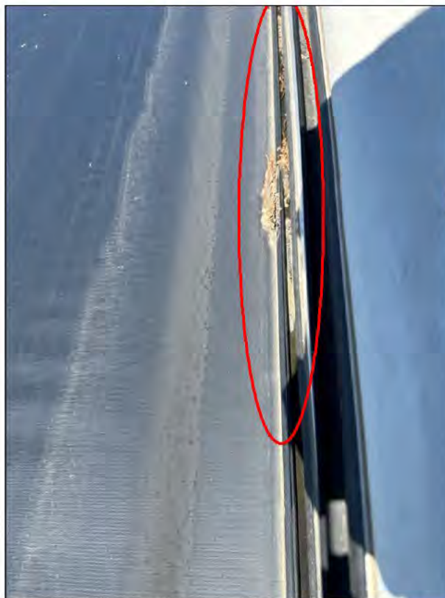
Front Curbside Awning Gutter from Top
