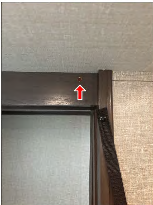
Bathroom doorway, rear
