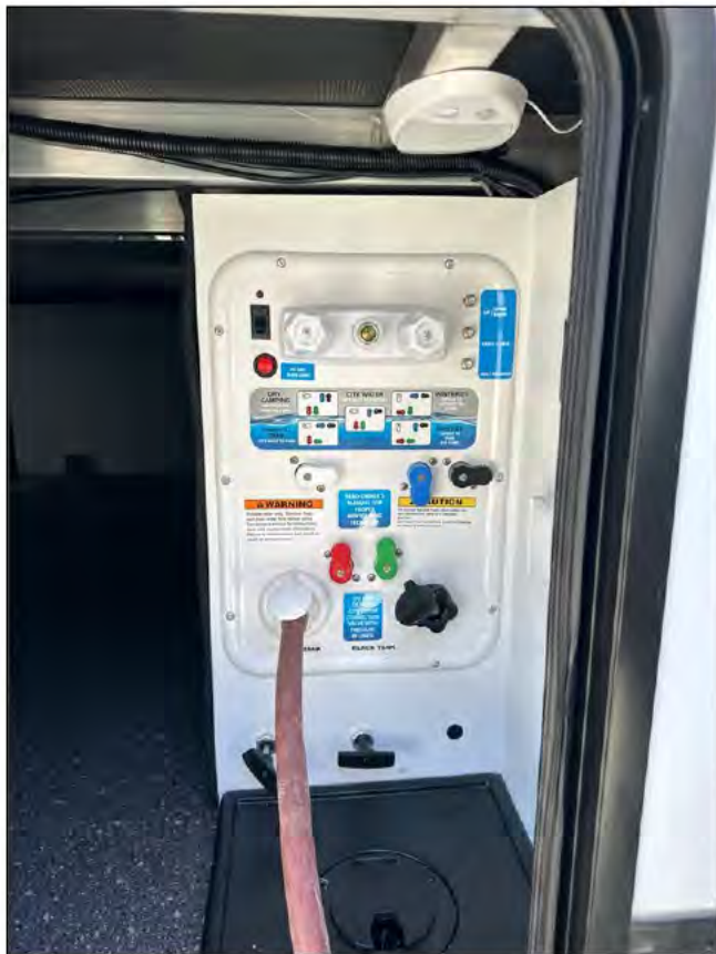
View of Water Controls from Streetside
