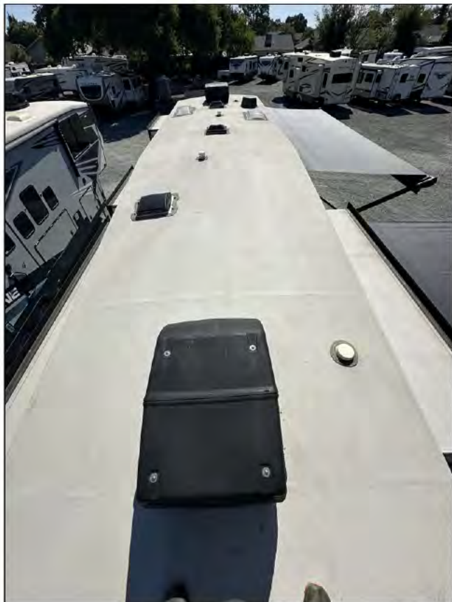
Roof (Rear to Front)
