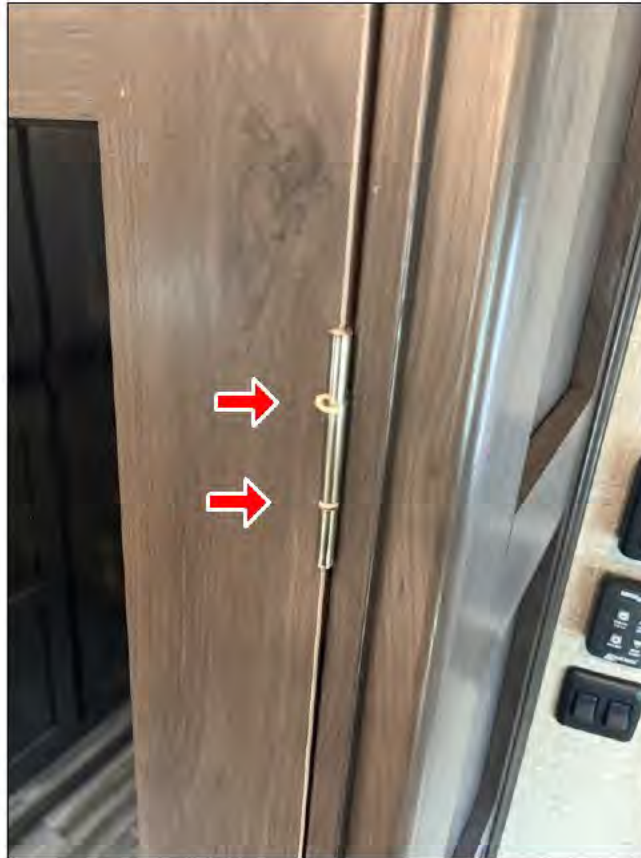
Curbside, top pantry door hinge
