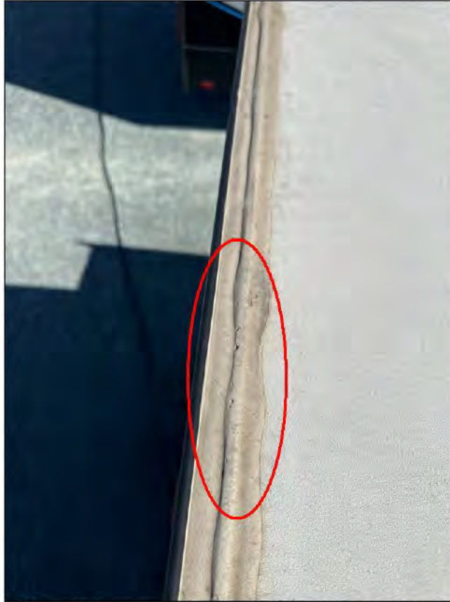
Top rear cap sealant toward middle (from top curbside)
