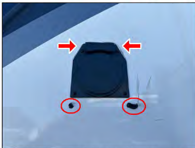
Dryer vent cover at top front of the streetside sidewall (from below)
