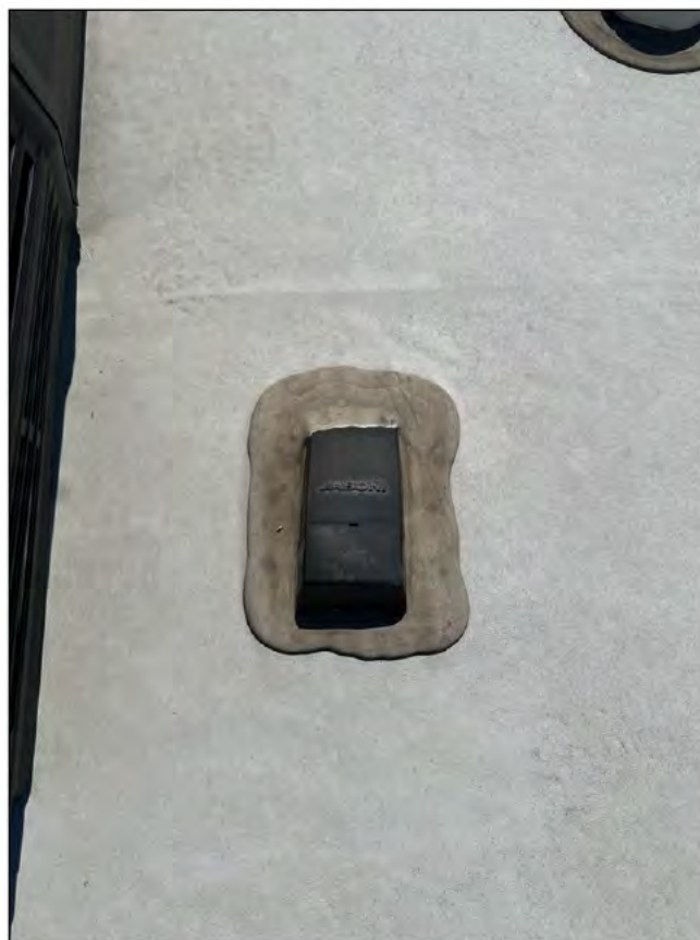
Solar prep connection on roof
