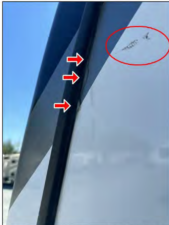
Streetside sidewall just rear of front cap toward roof
