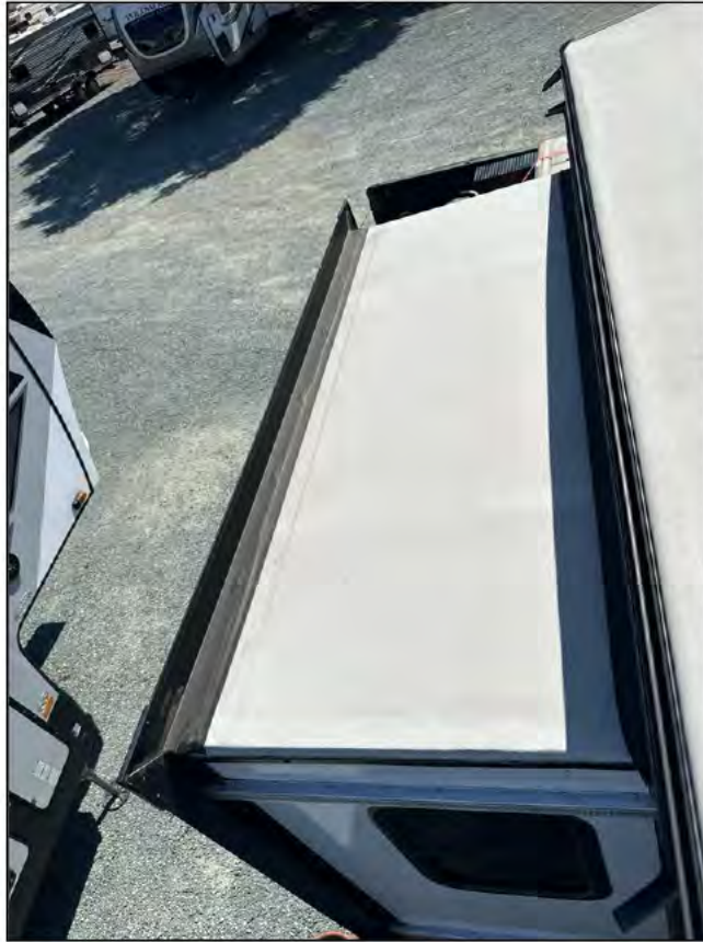
Streetside front slide roof from rear
