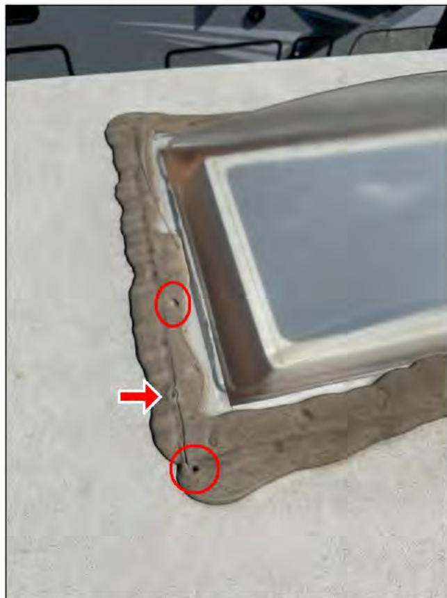
Streetside skylight from rear curbside corner
