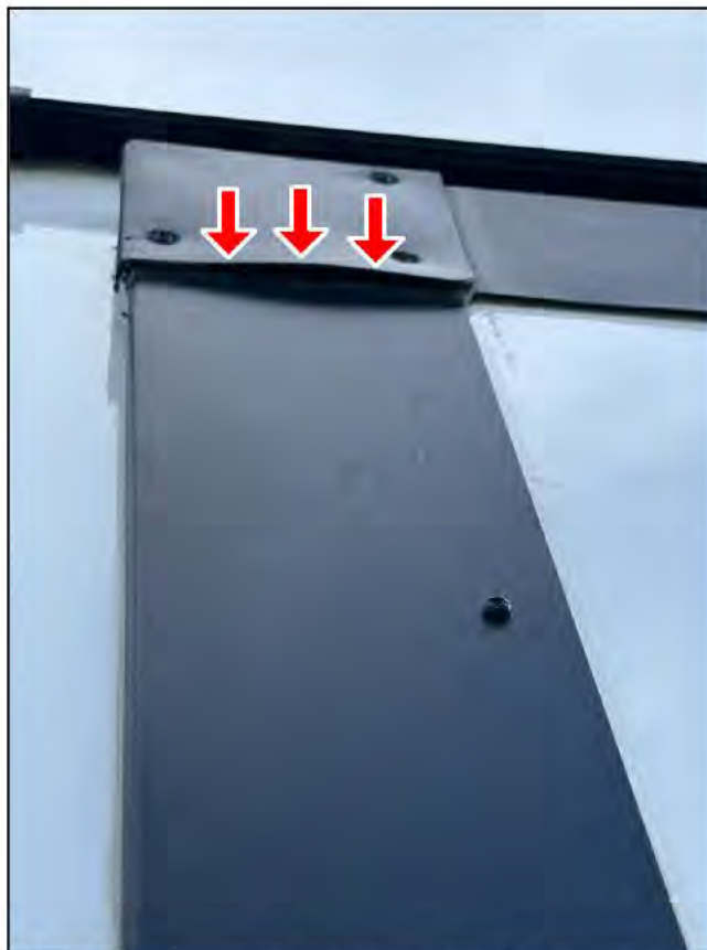
Top front corner of the streetside center slide (from bottom)
