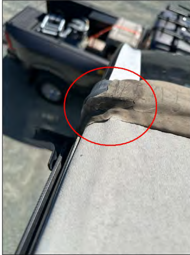
Front streetside roof seal
