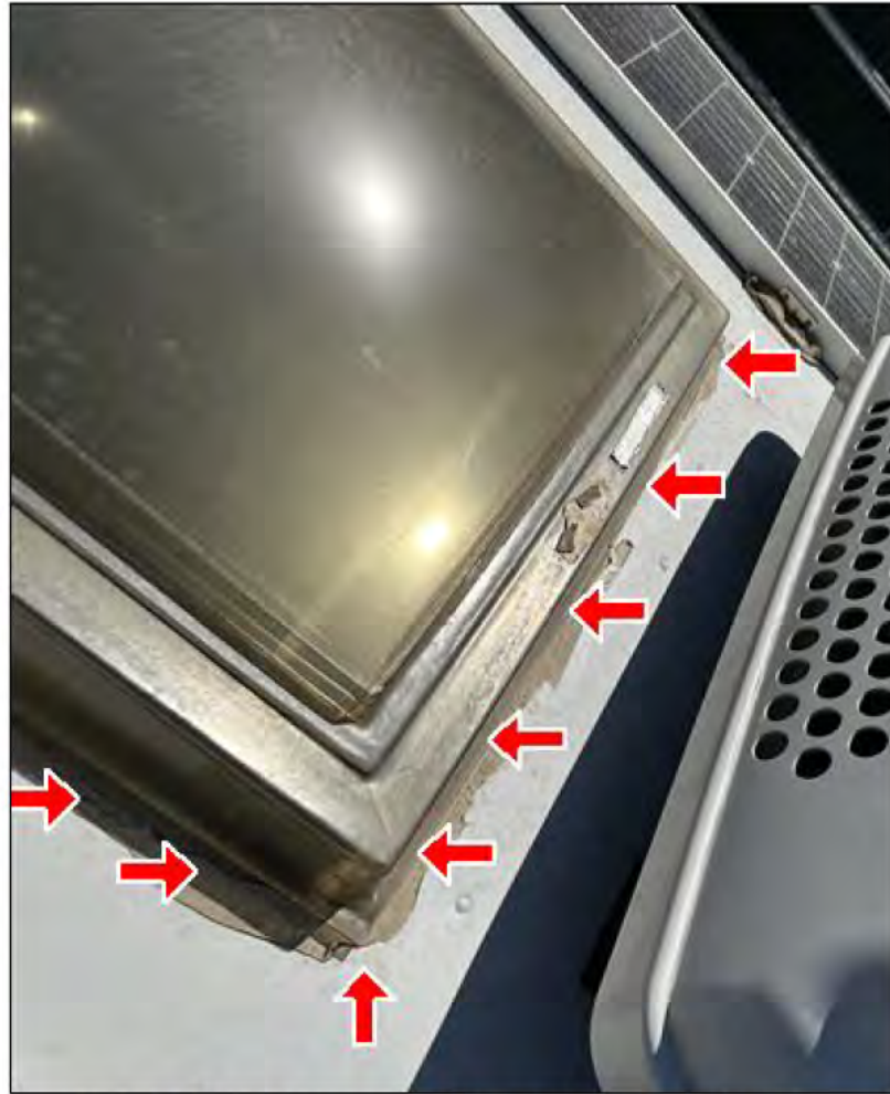
Curbside front corner and front edge of skylight (from curbside)
