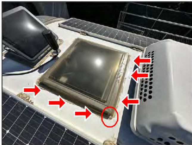
Curbside and front edges of skylight (from curbside)
