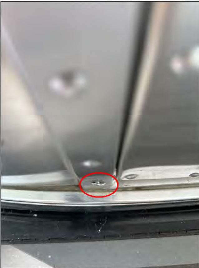
Rear bottom view of rear cap streetside (close up from top)
