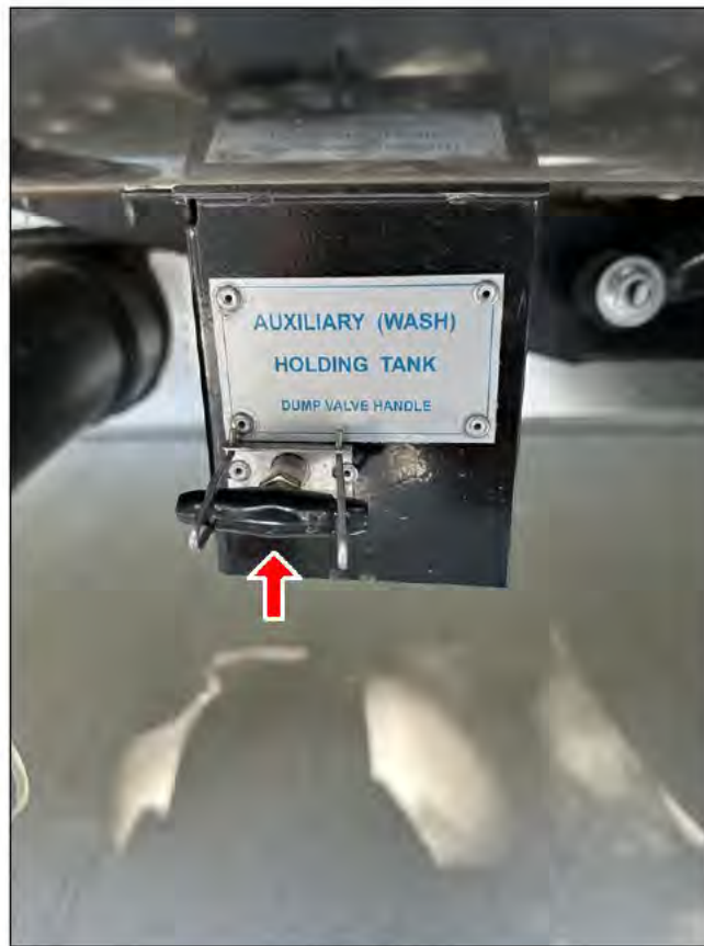
Gray tank dump valve handle on streetside toward front
