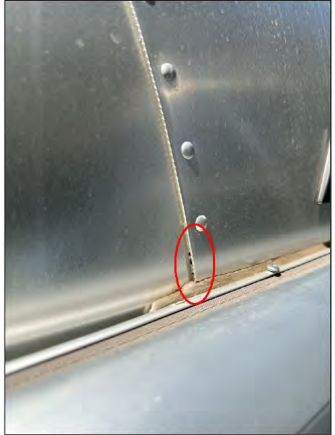
Top rear streetside seal (close up)
