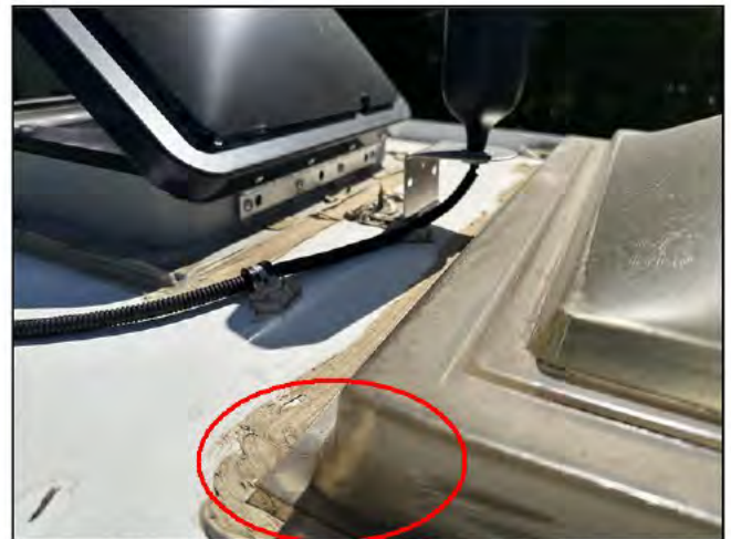
Curbside rear corner of the skylight
