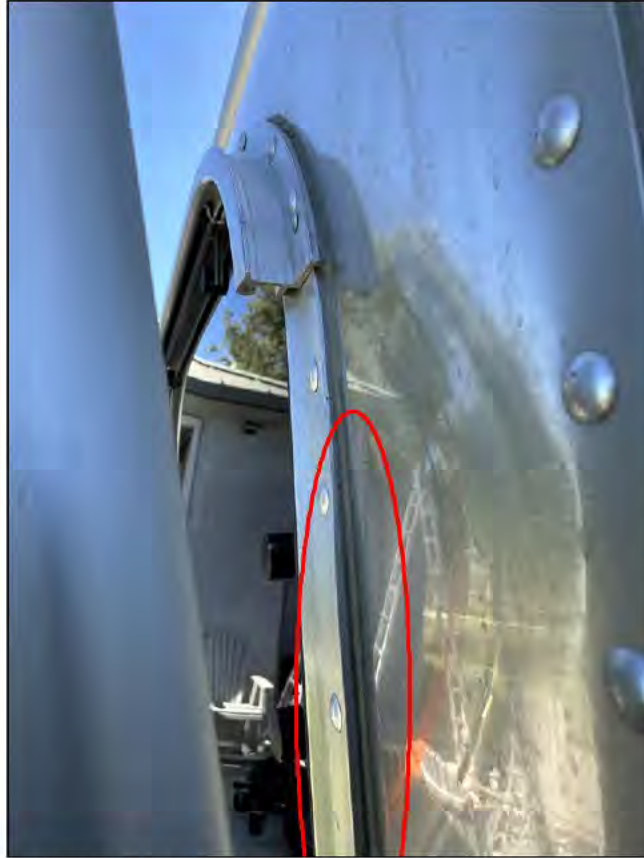
Curbside front window just rear of front awning arm
