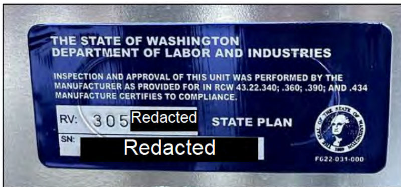
WA State Department of Labor and Industries Inspection Sticker
