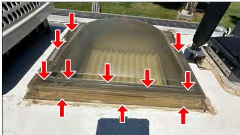
Skylight on rear end of roof from streetside
