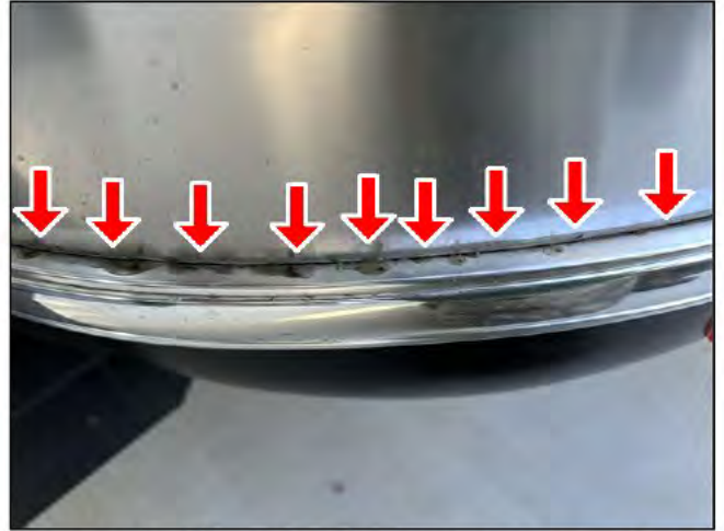
Rear/curbside wall behind curve at rear (close up)
