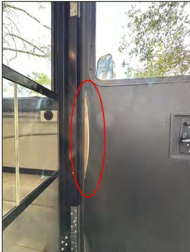
Middle front edge of main door
