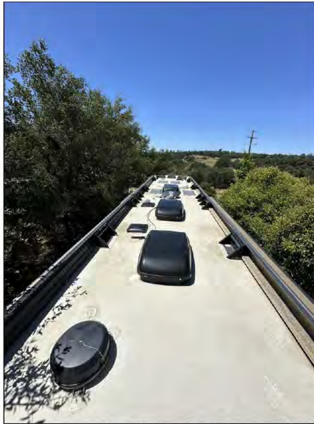
Roof (front to rear)
