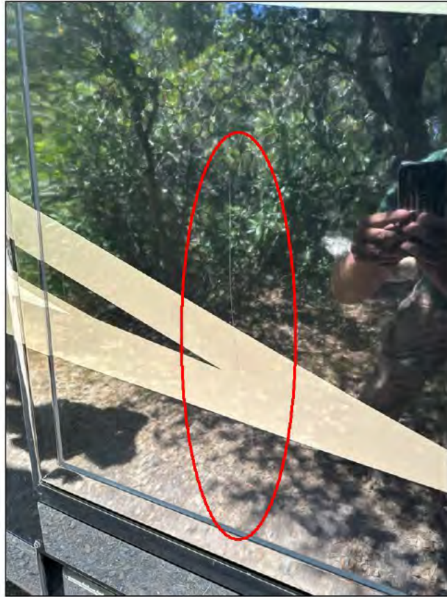
Bottom middle of main door
