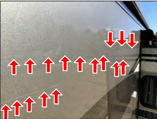
Upper curbside side wall forward of rear wall
