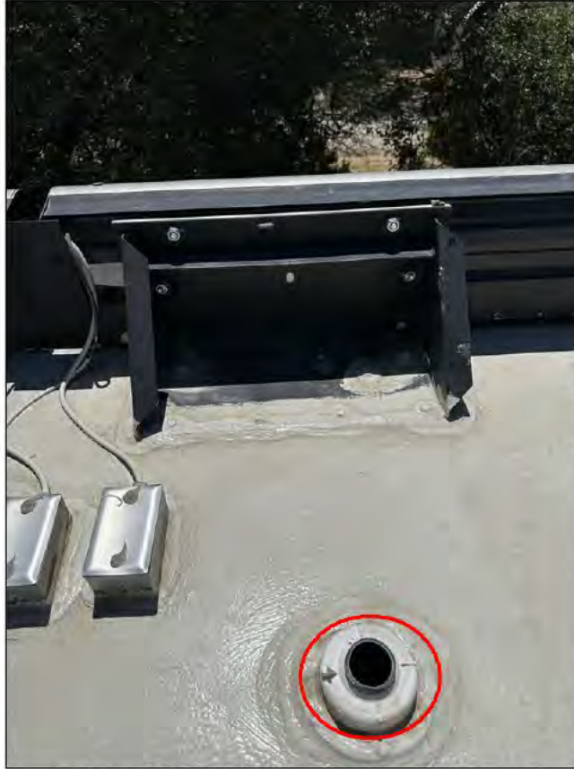
Curbside roof between rear and center AC units (from streetside)
