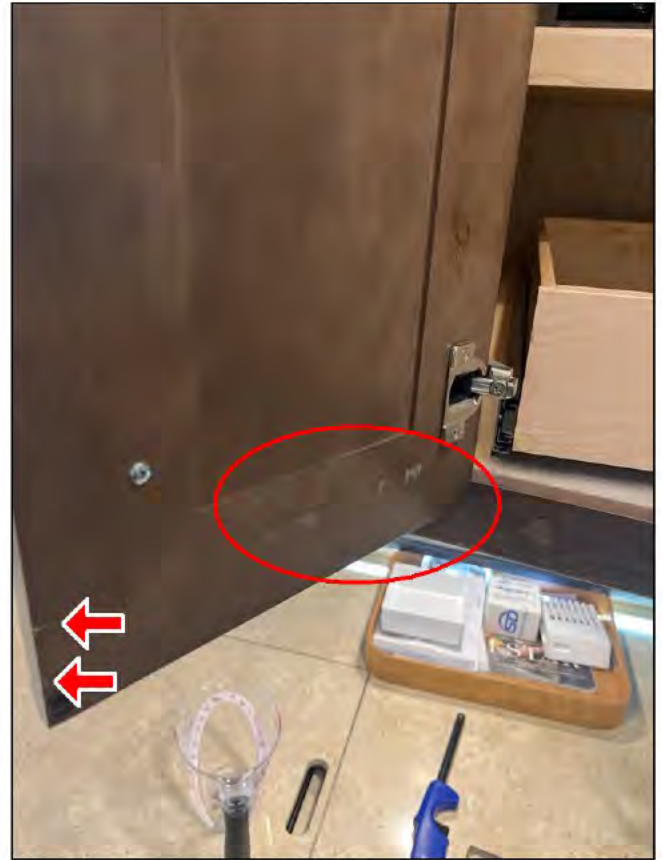
Front curbside cabinet door above kitchen sink
