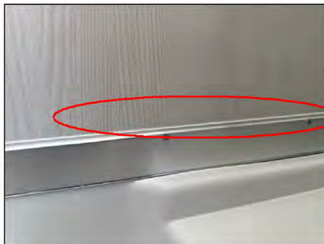
Streetside wall at bottom of bathroom (close up)
