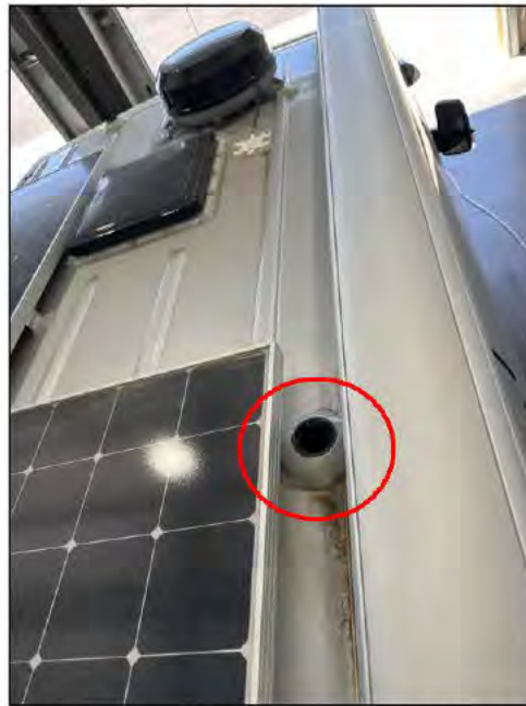
Curbside roof above sliding door
