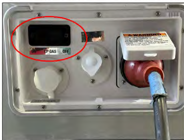
Streetside water and power bay with LP gas switch
