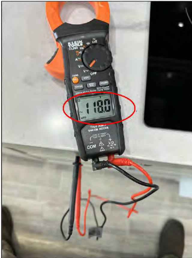
Generator voltage under load at kitchen outlet forward of cooktop
