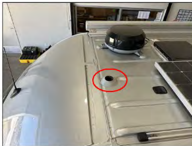
Front center of roof
