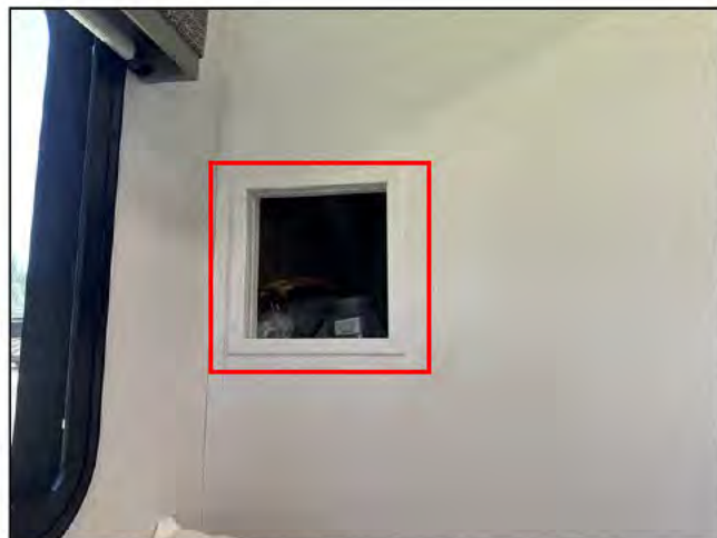
Close up of wall on streetside separating bedroom from living area
