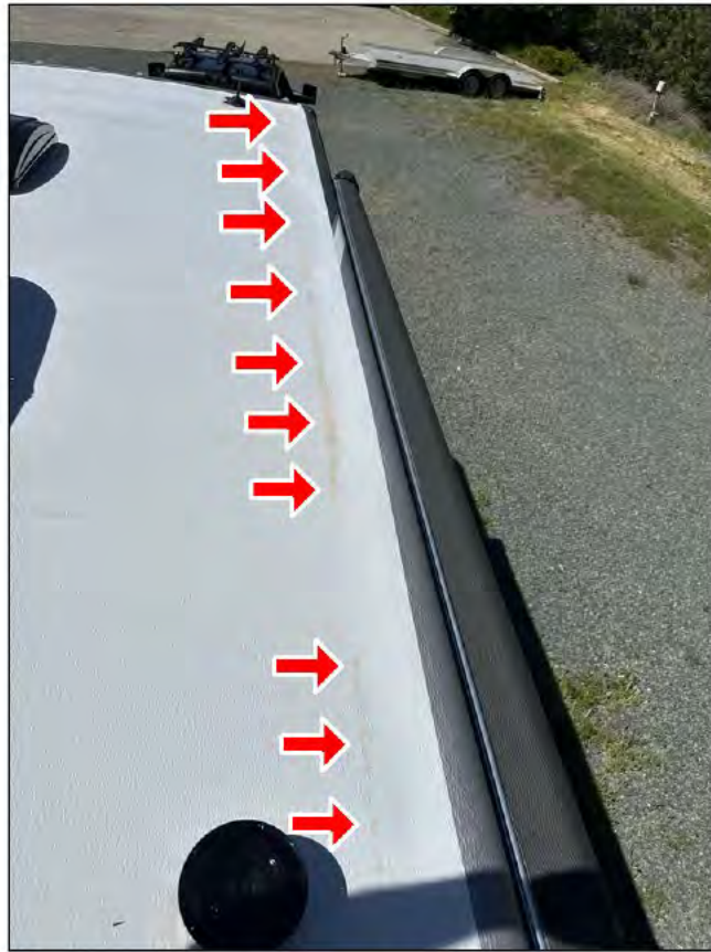
Curbside edge of roof from rear to front
