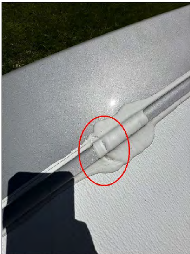
Middle of rear cap seam from front curbside
