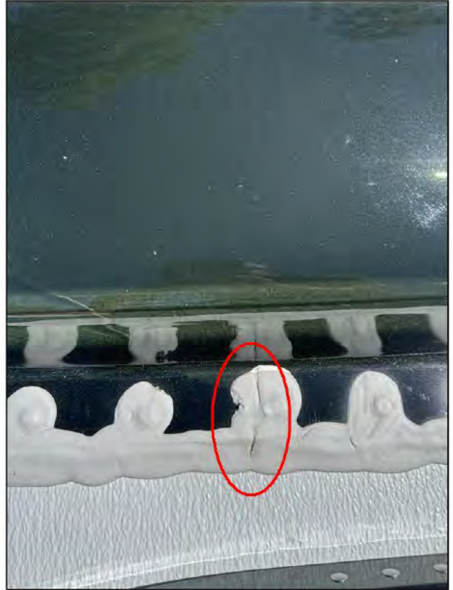
Close up of front edge of rear skylight (front to rear)
