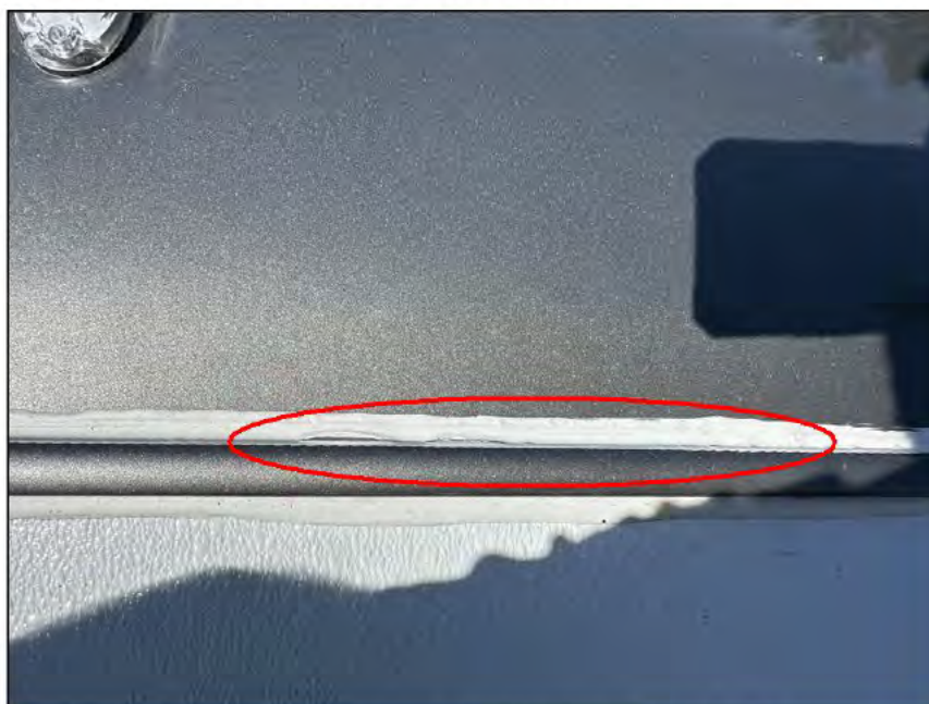
Close up of front cap seam toward curbside
