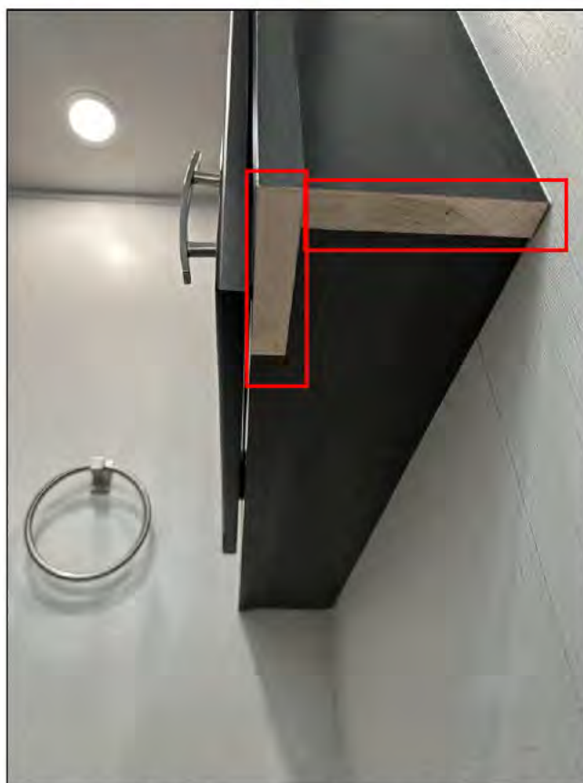
Bottom of bathroom medicine cabinet (from shower side)
