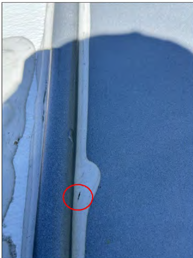
Close up of rear cap seal at middle (from streetside)
