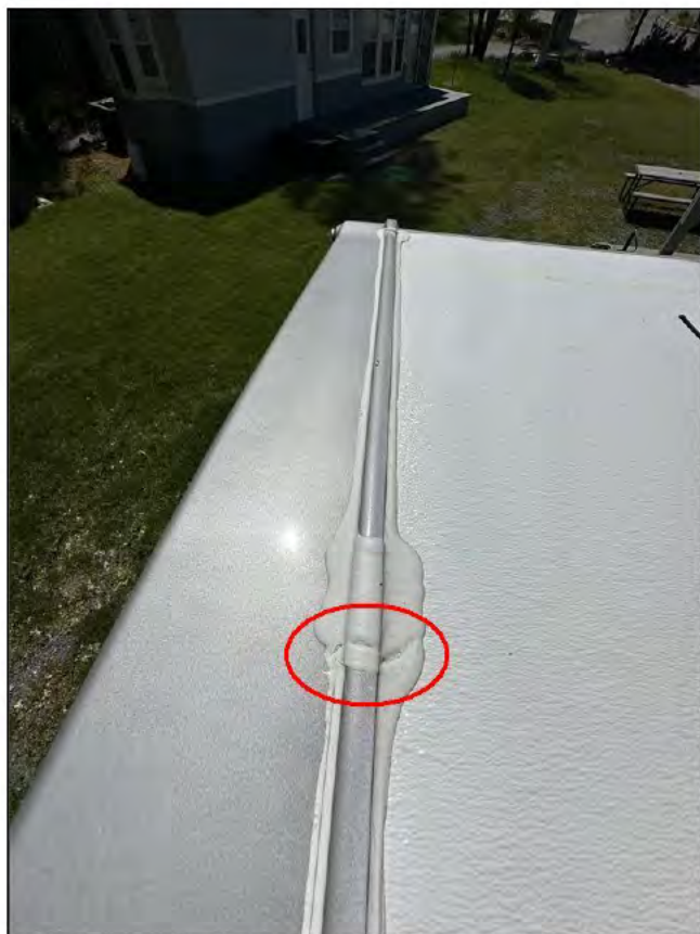
Middle of rear cap seam from curbside
